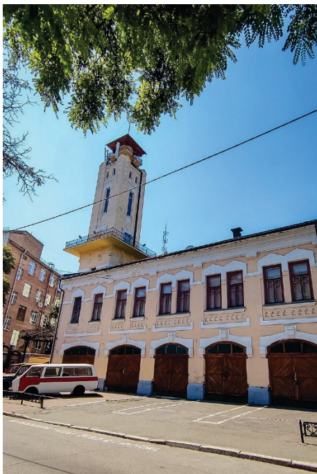
Fig. 2. Ukrainian National Chornobyl Museum. The former depot building of the Podil Fire Department, Kyiv [5]
