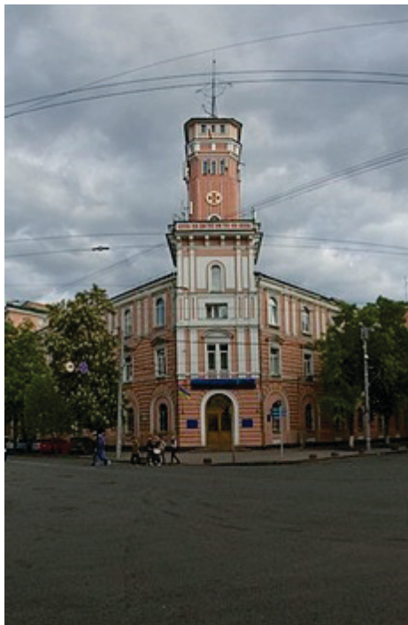
Fig. 1. The Main Office of the State Emergency Service of Ukraine in Kyiv. The former depot building of the Starokyiv Fire Department, Kyiv [3]
