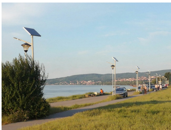
Fig. 12. Solar Lighting at Ada Huja in Belgrade, 2011
